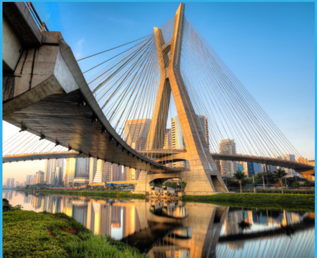
Estaiada Bridge, Sao Paulo, Brazil
